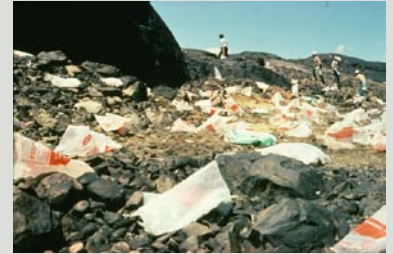
Workers spreading lime and fertilizer on barren lands in Copper Cliff area.
